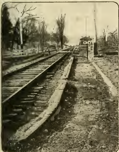
SECTION OF THE ANCIENT SUPER-STRUCTURE
